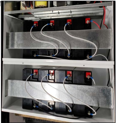
Battery brackets installed on the front
